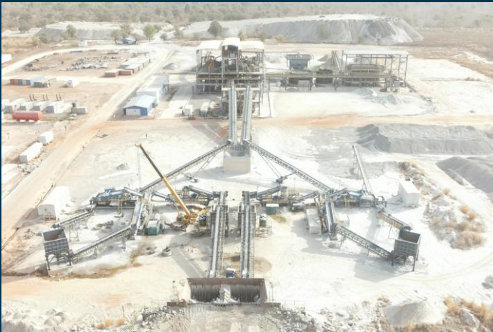
Stage 1 Dense Media Separation (DMS) plant
