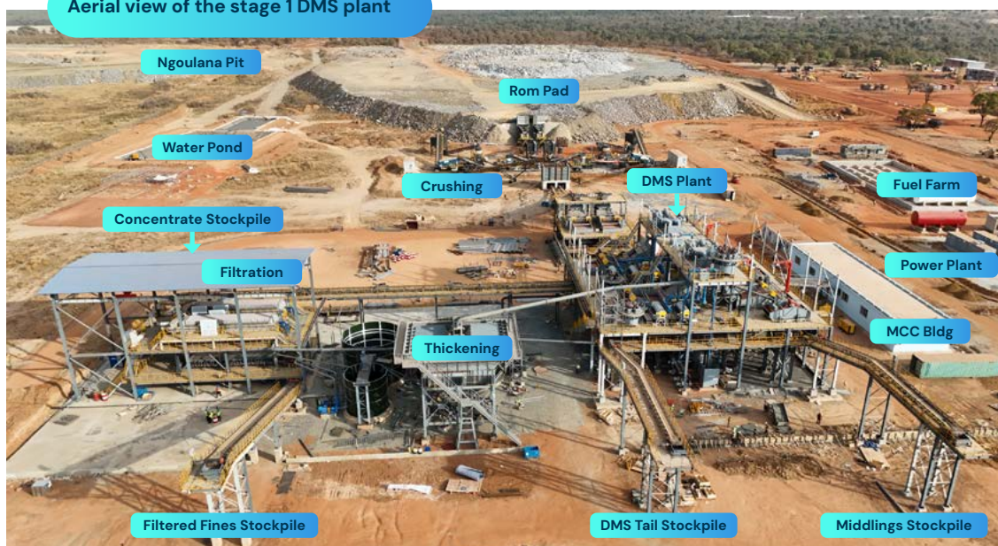
Aerial view of the stage 1 DMS plant
