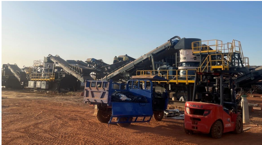
Assembly of secondary and tertiary crusher modules
