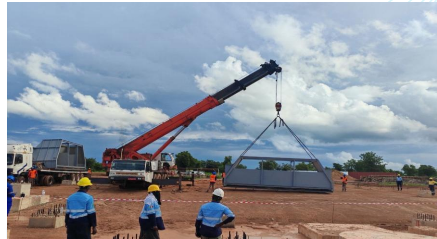
Offloading platework on site
