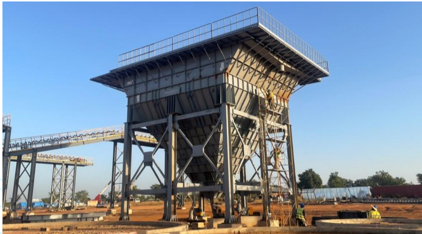
Plate style thickener assembly
