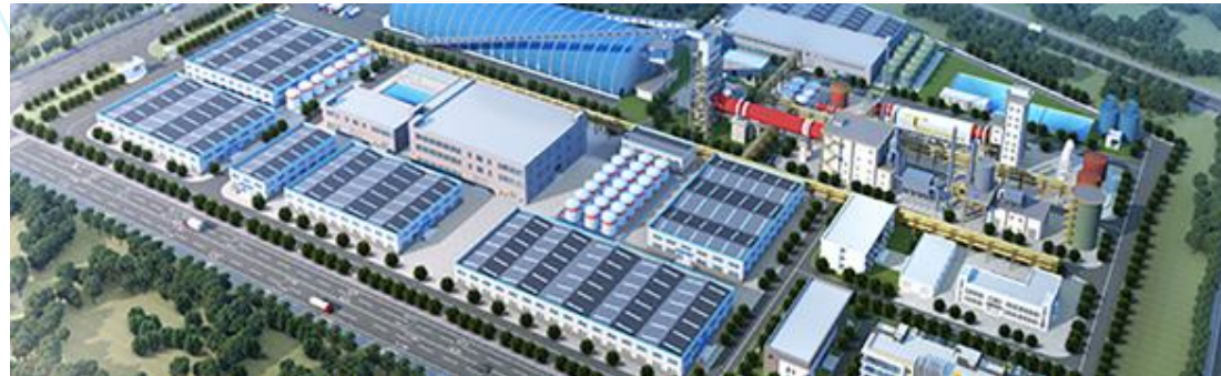
Hainan Mining's battery-grade Lithium Hydroxide Plant in Hainan Province, China
