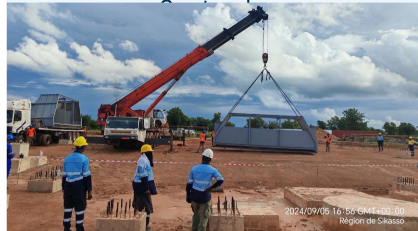
Crusher chute offloading – 5 September
