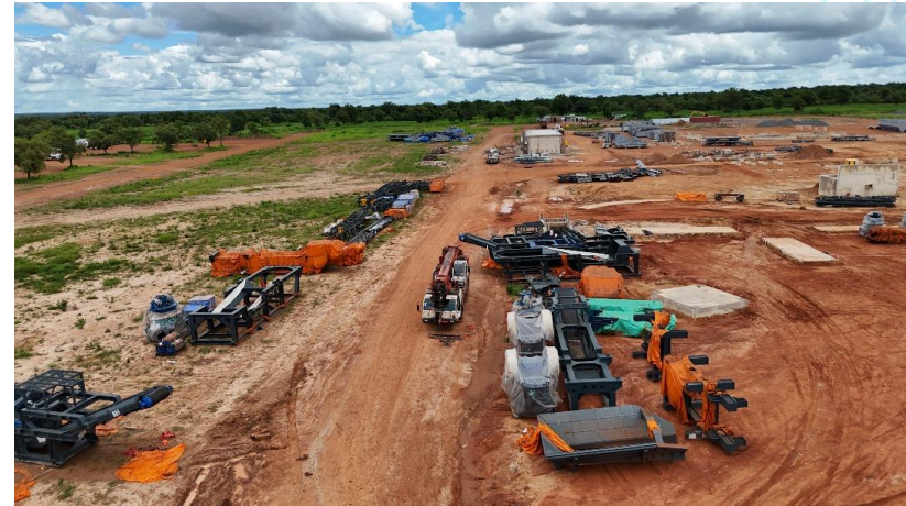
Crushing Equipment on site – 23
