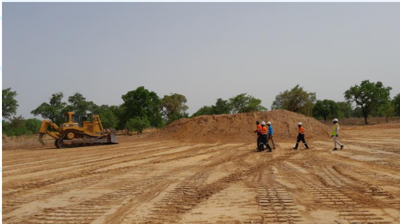
Top soil stripping Plant Site
