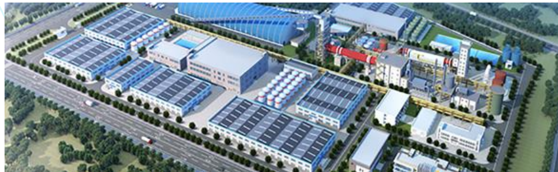
Hainan Mining's battery-grade Lithium Hydroxide Plant in Hainan Province
