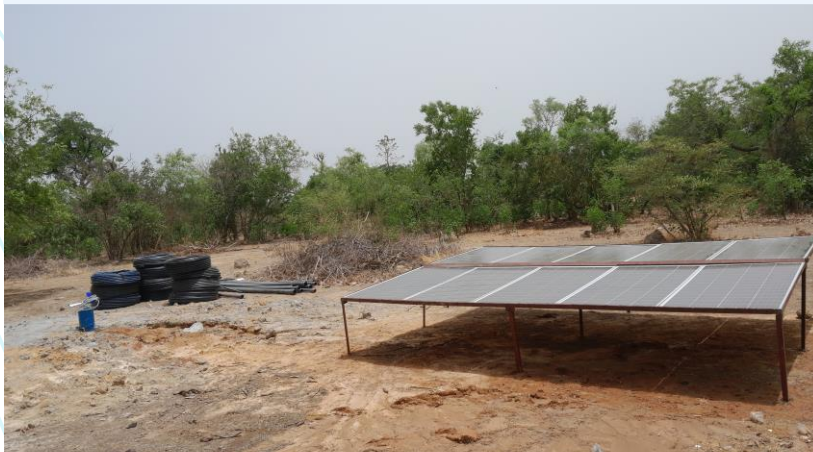
Solar powered bore pump installation
