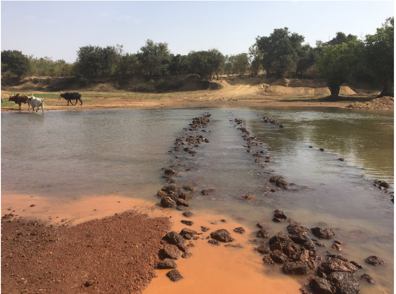
Baoule River – Bougouni Project
